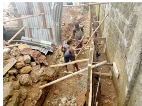
Working to put up the zinc panels
